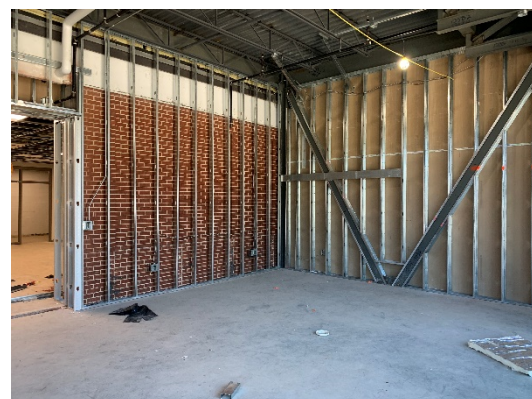
Level 2 Existing to New Addition Framing
